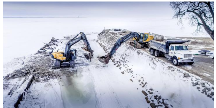
When the ice hits 18 inches thick, even a 40,000+ pound excavator can roll right out onto the lake.
