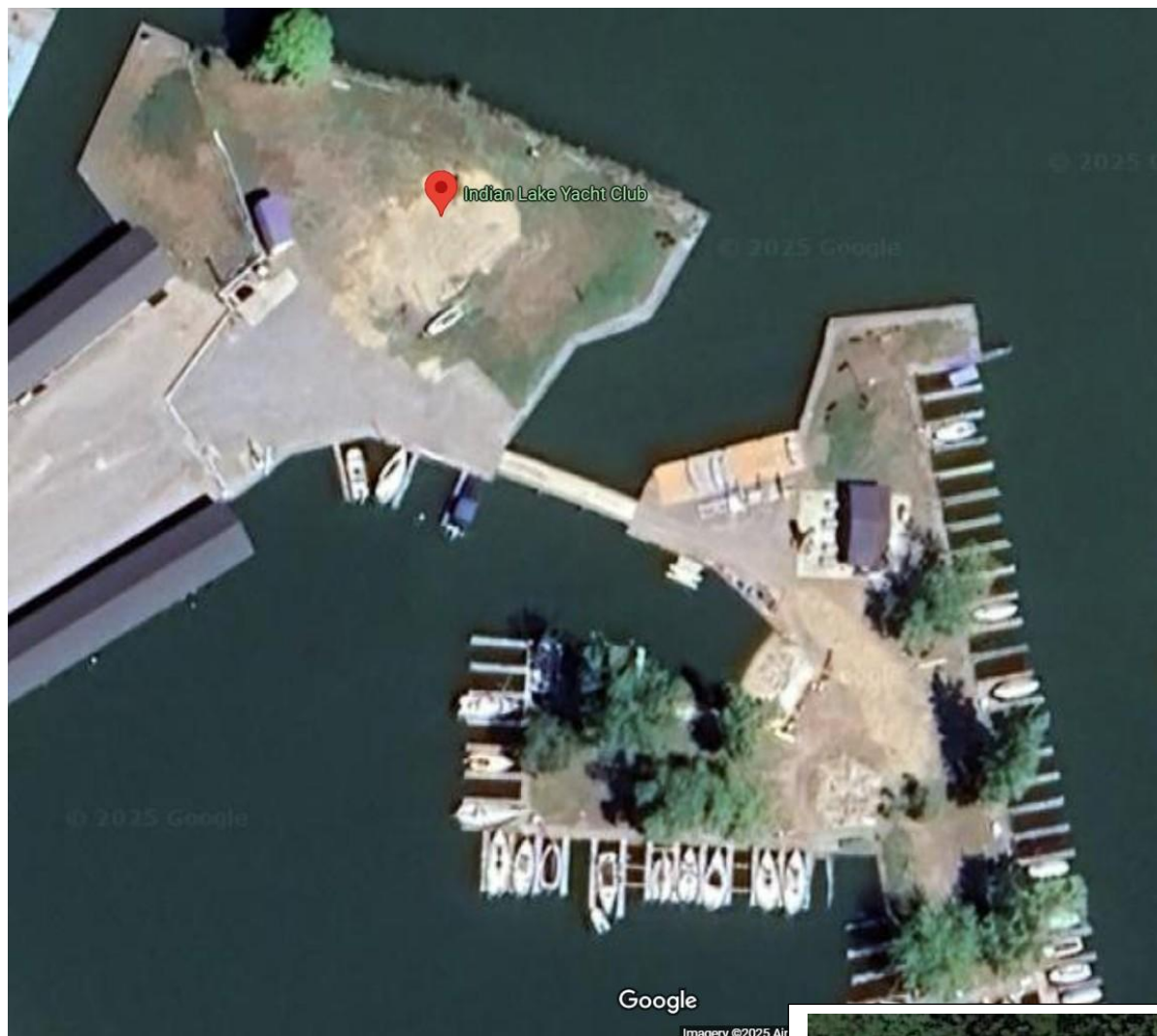
Satellite view of Indian Lake Yacht Club after all the tornado debris was removed but before any of the materials for the new club house are delivered
