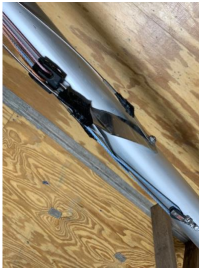
spin hoist block & all taped up.
