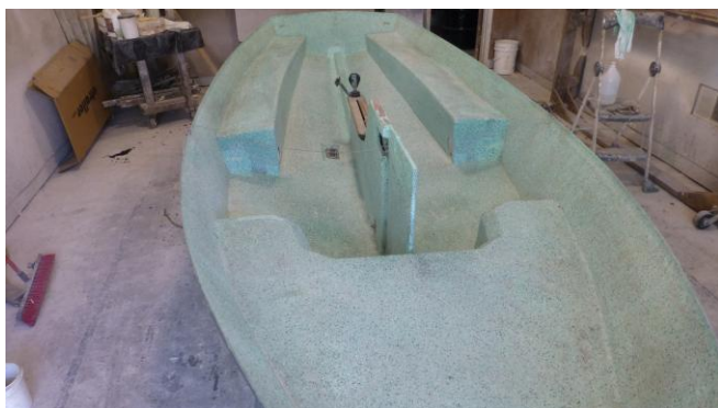
Interior of an old hull finally ready to be mated with a new deck. Note virtually every piece of hardware has been removed (time and money)
